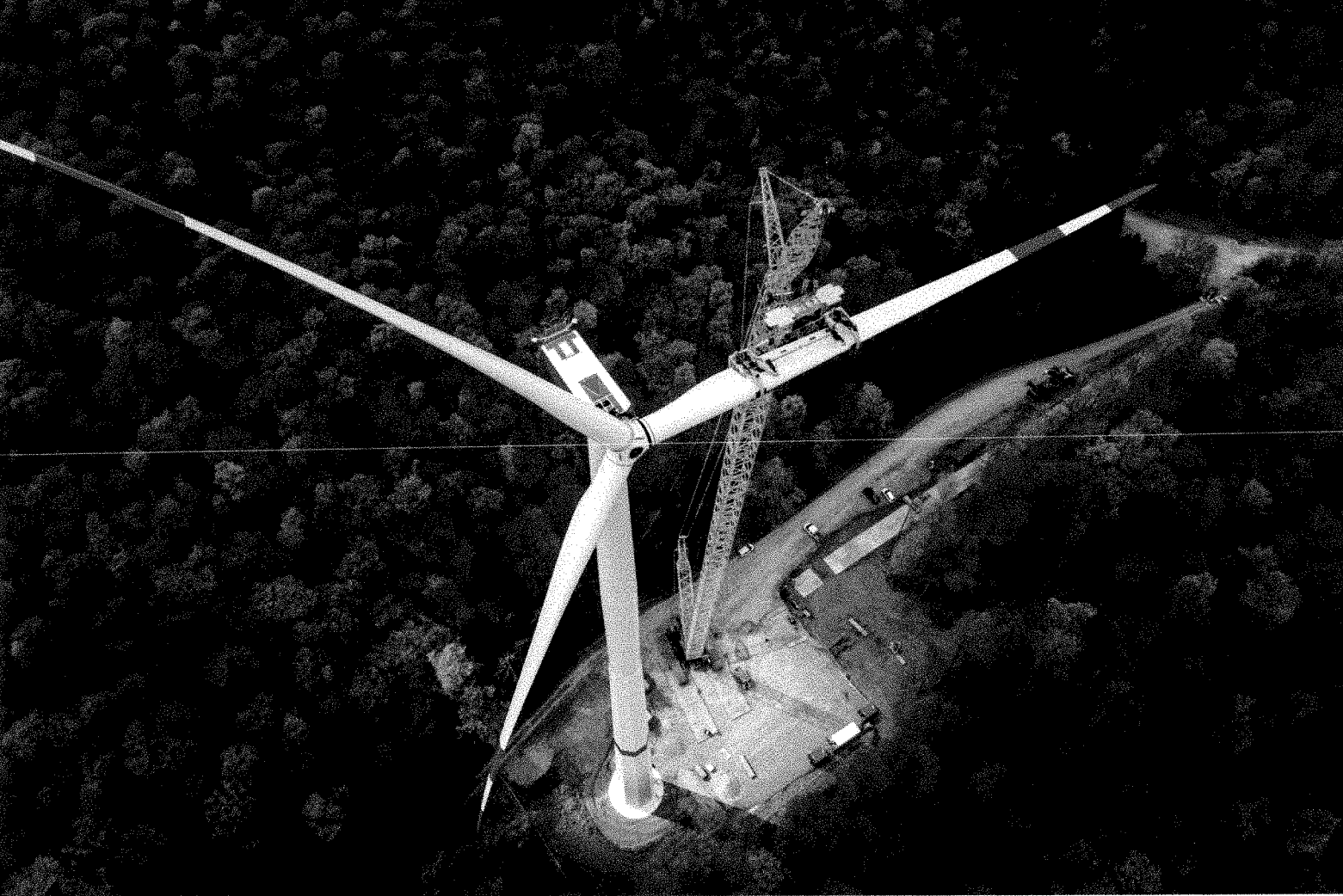
Aerial view of wind turbine under construction. Credit: P. Heitmann/Shutterstock
